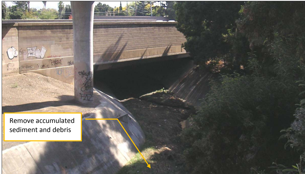
Figure 3-12 I-680 Bridge (Looking Upstream)
